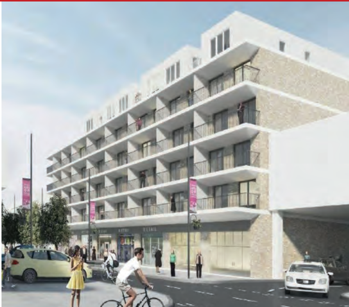
One of Crawley's new town centre residential developments
