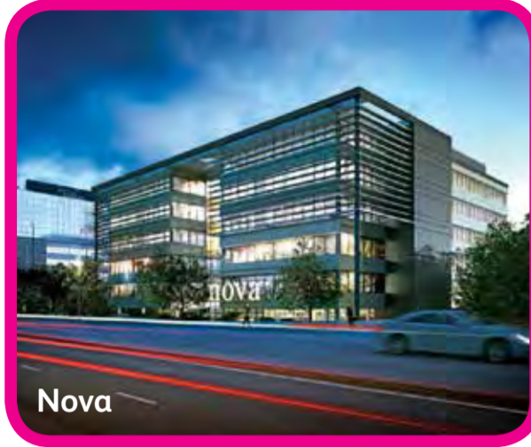
Nova London Road and County Oak Way junction improvements
